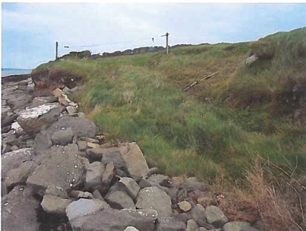
Figure 6: Means of access to foreshore to west of outfall pipe
