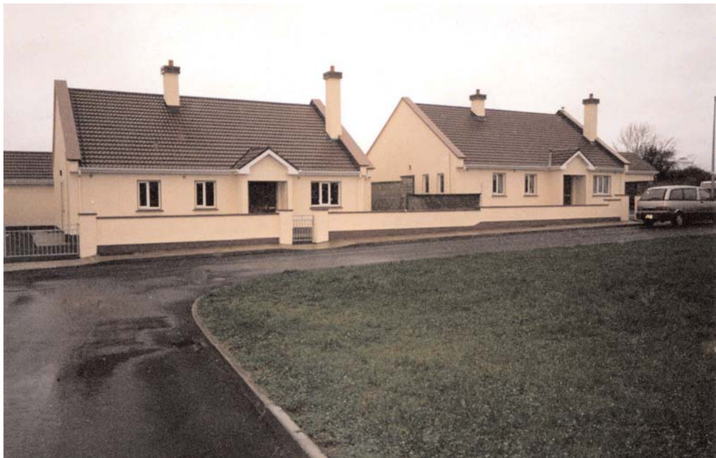
Cloonlyon Crescent, Ballygar, Co. Galway
